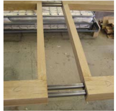
The two ends joined by sliding tubes, open
